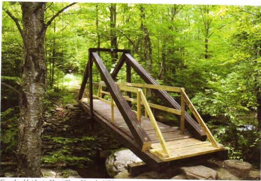
Completed bridge in Platte Clove. Photo by Jeff Senterman
